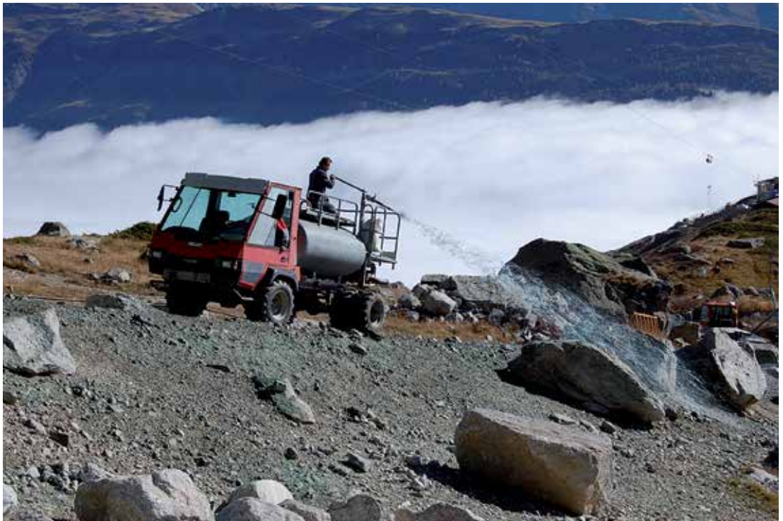
Figure 39 - Hydroseeding of the experimental plot at Courmayeur - Pavillon.
